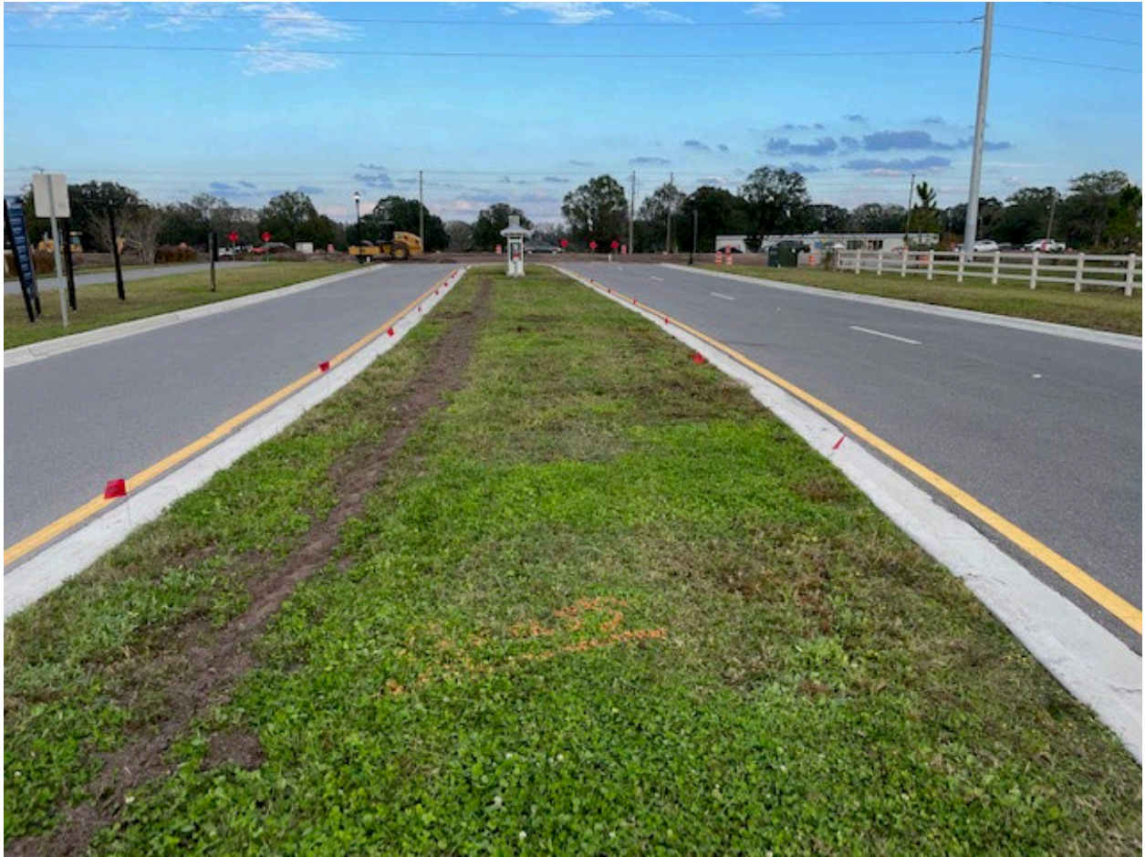
Irrigation lines have been lain in the median at the end of Grand Live Oak Blvd.
