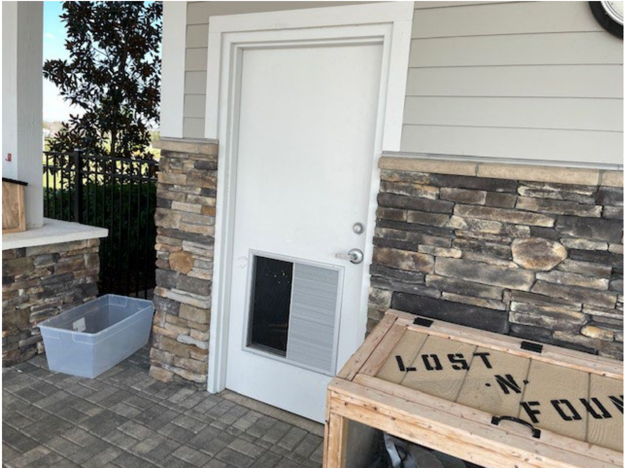
The door for the storage closet needs a new vent grate.
