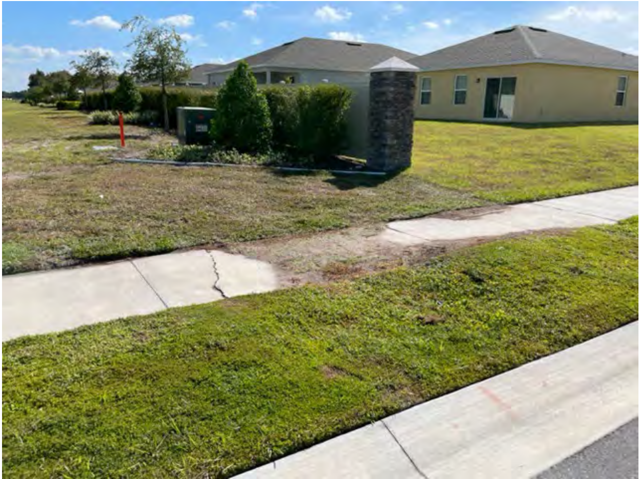
Sidewalk is sinking at Gliding Eagle Way and Grand Live Oak Blvd. Collecting quotes for repair. Pipe laying on ground has been removed.
